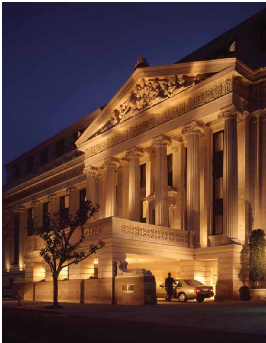
Four 60kW Capstone microturbines provide cooling, heating, and power to the prestigious Ritz-Carlton hotel in San Francisco.
